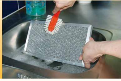
3. Wash the vent from inside and outside using a brush and detergent. The space between the regulative part and the neck must be kept clean as it affects performance of the vent. Dry the vent. Note: Do not twist the regulative part in the centre! It has been locked during the ventilation check up to ensure that the exact amount of air is ventilated
