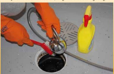
4. Wash the protective grid from both sides and place it back. Make sure that clean water was left inside the drain to prevent sewer gas coming into the room air.
